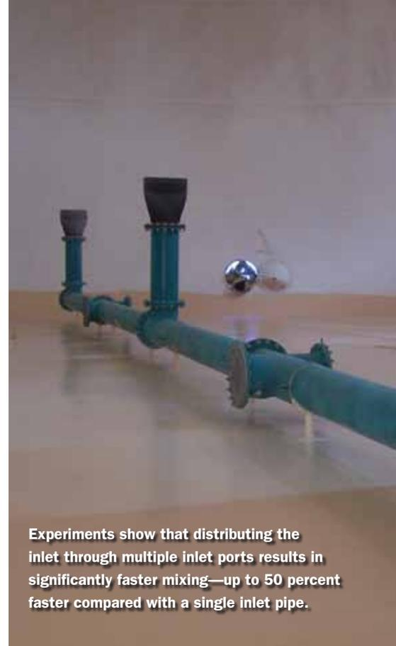
Experiments show that distributing the inlet through multiple inlet ports results in significantly faster mixing—up to 50 percent faster compared with a single inlet pipe.
