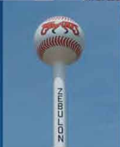
200,000 Gallon Zebulon, North Carolina
