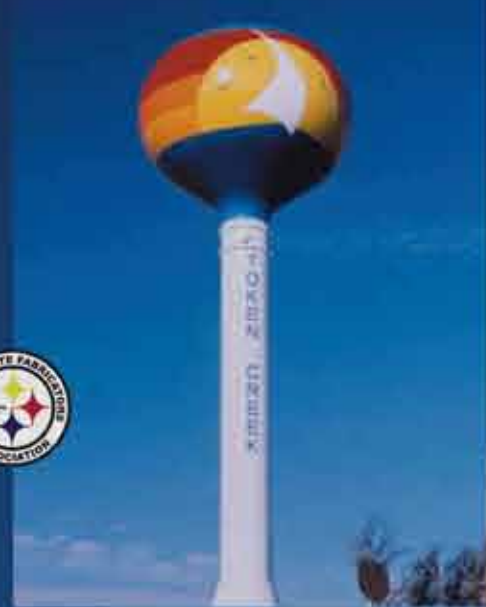
200,000 Gallon Burke, Wisconsin Steel Tank of the Year 1995 - Steel Plate Fabricators Association
