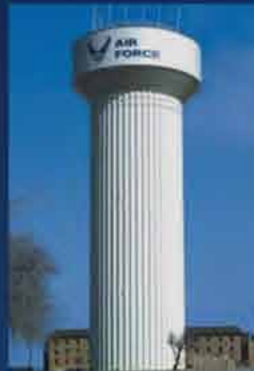
1,000,000 Gallon McConnell AFB, Wichita, Kansas
