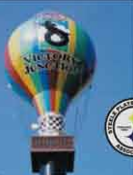
150,000 Gallon Randleman, North Carolina Steel Tank of the Year 2004 - Steel Tank Institute/Steel Plate Fabricators Association
