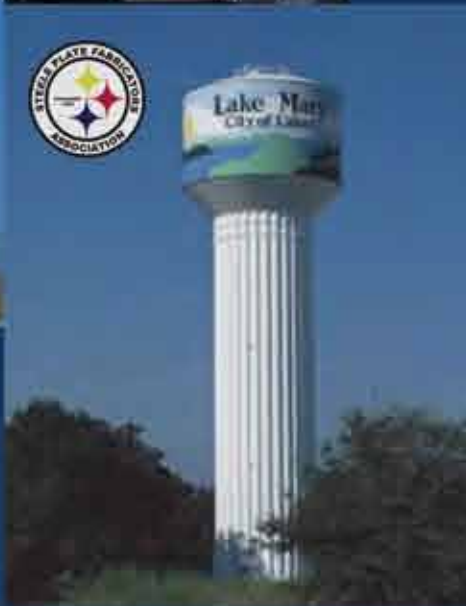
500,000 Gallon Lake Mary, Florida Steel Tank of the Year 2002 - Steel Plate Fabricators Association
